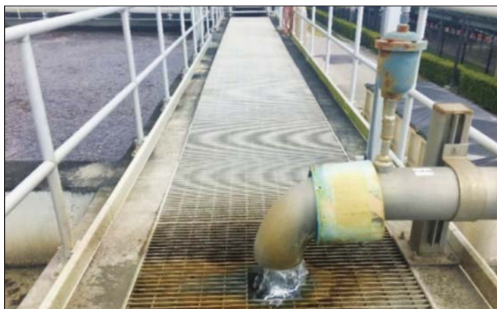
Figure 1. Photo of Point of Reverse Osmosis Concentrate Discharge to Aeration Basin
